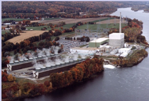
Vermont Yankee Power Plant (AP file photo)
